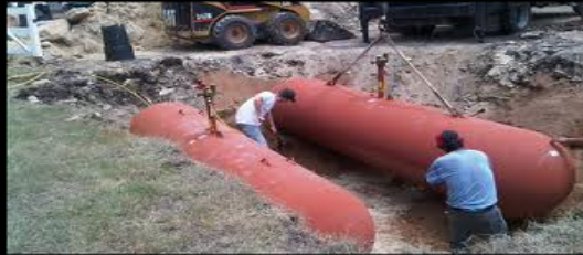
1000 Gal Underground Tank Installation
