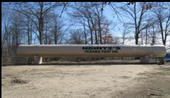
18,000 Gal Bulk Storage Facility (transport delivery)
